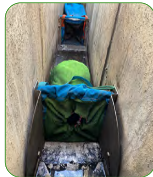
Frontline™ TDI trench drain filter inserts
