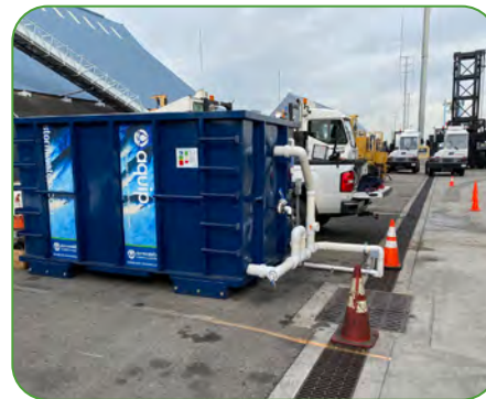
Trench drain with Frontline™ TDI filter inserts (not visible). Aquip 50 downstream of TDI.
