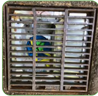
Frontline™ CBI 100 filter element in an adjustable frame (L), and under an existing catch basin grate (R).
