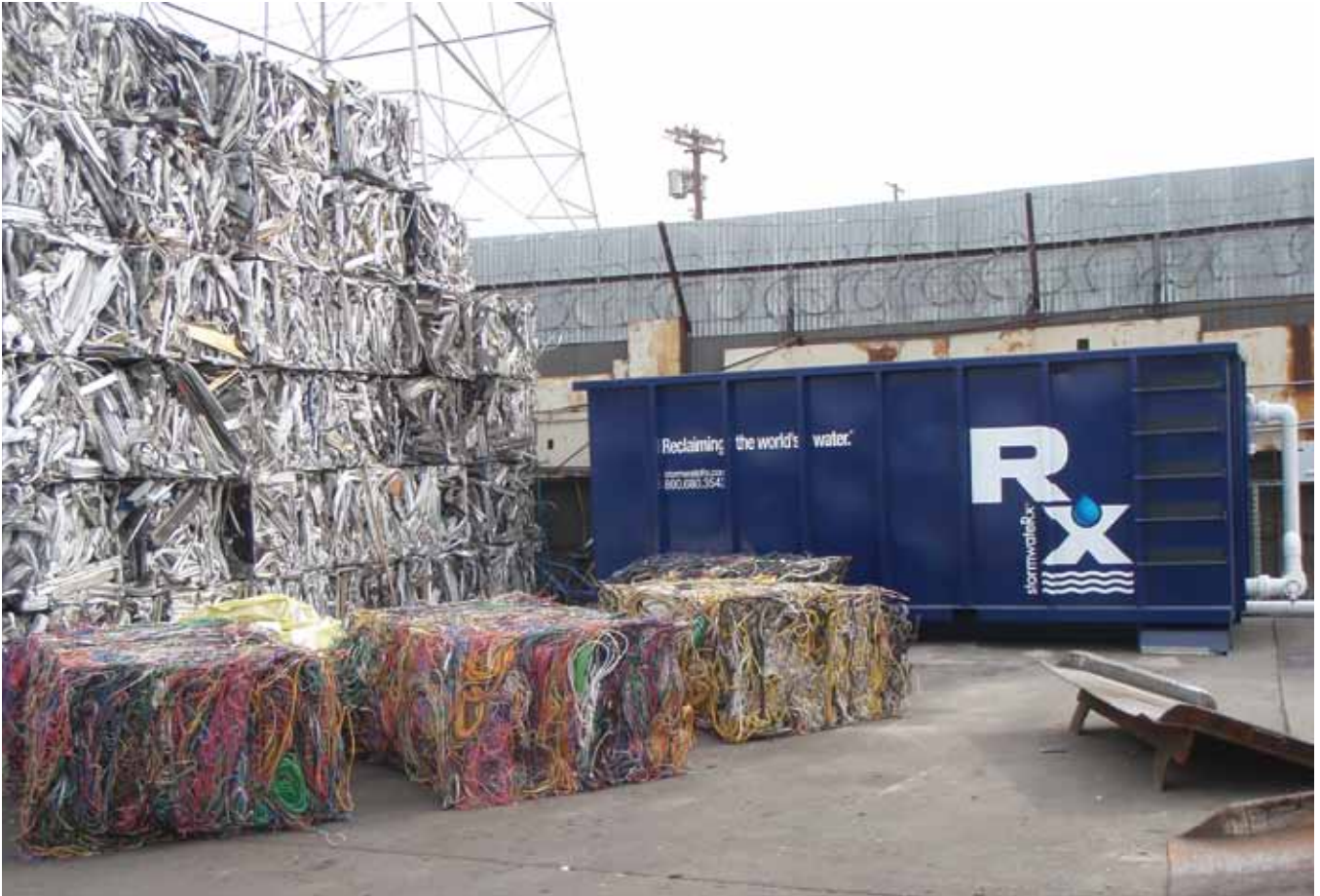
Above is shown an Aquip stormwater filtration system for surface water discharge from an industrial site.
